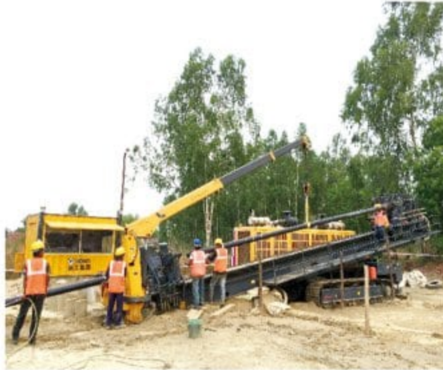
XZ3000在印度坎布尔穿越恒河2.2公里 XZ3000 HDD works to get through Ganga River by 2.2Km Kanpur
