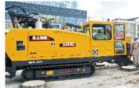
XZ450水平定向钻机在上海施工 XZ450 HDD working in Shanghai
